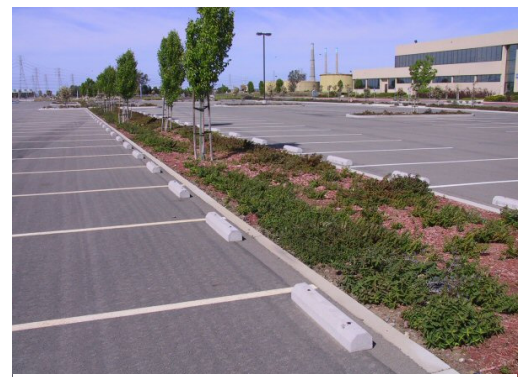
Swale designed to receive runoff from paving on either side
