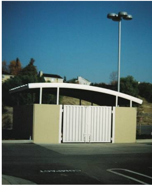
Roofed and bermed refuse area.
