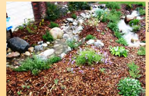
Overflow from the rock-lined swale flows to a rain garden that drains within 48 hours (shown in March 2011).
