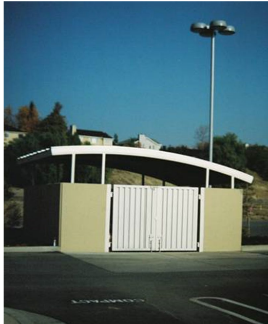
Figure 3.1. Roofed and bermed refuse area.
