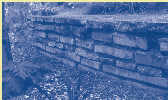
Broken concrete is used to create a retaining wall.
