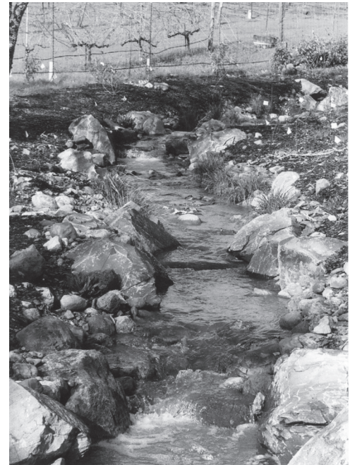
A series of boulder step pools in a restored channel.
