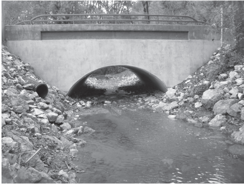
Arch culvert with natural stream bottom
