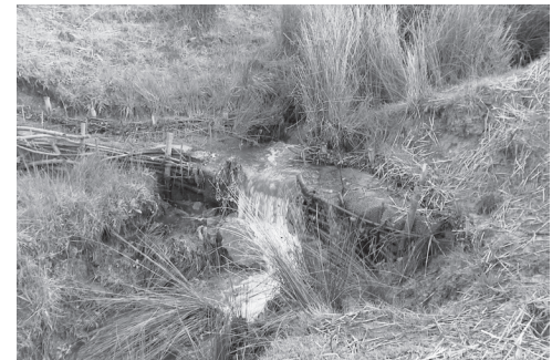
Willow wall headcut repair
