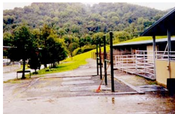
This horse wash area drains into a grass filter strip (along the row of trees). The filter strip traps sediment, horse manure and other contaminants.
