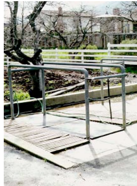
A curb directs horse wash water away from the creek. Keep horse wash water out of creeks, seasonal drainages, and storm drains. Horse wash areas should be kept clean of manure and grooming products.
