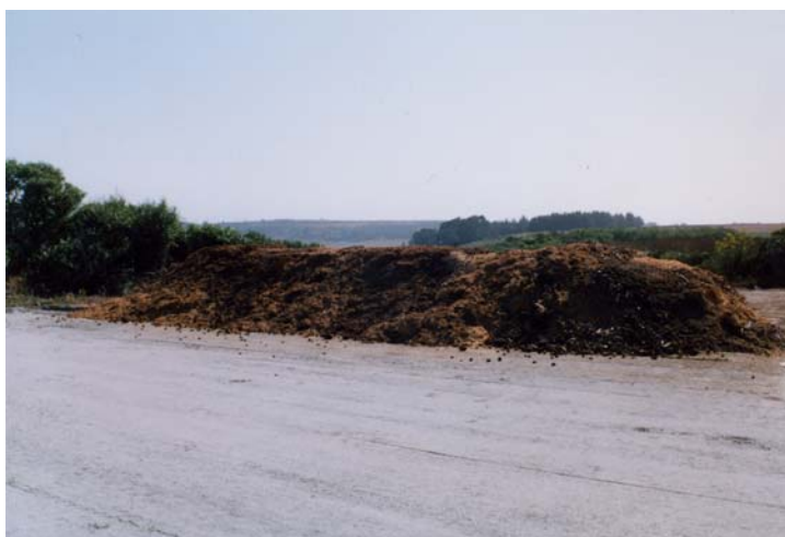
An impermeable surface, graded to control runoff.
