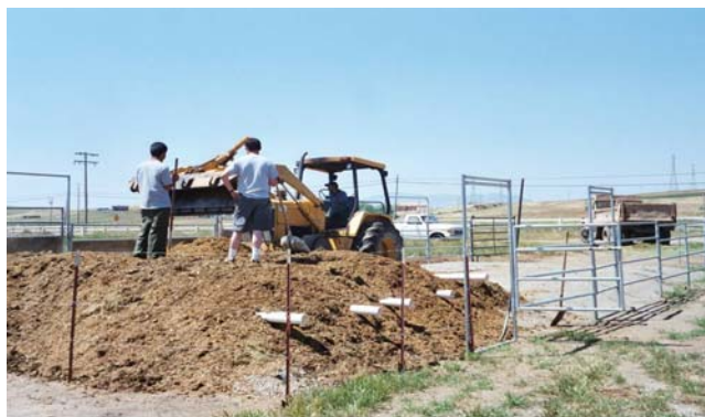
This compost method uses perforated pipe to bring air into the center of the windrow. Portable fencing keeps cattle out.
