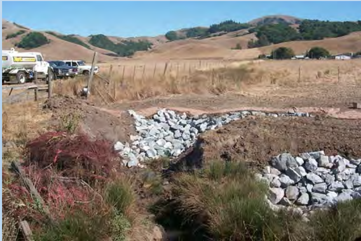
During (showing grade stabilization)
