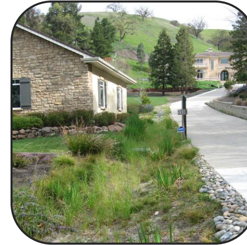
Large Residential Rain Garden
