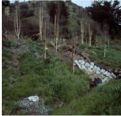
Grassed drainage area.
