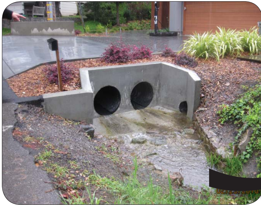
RUNOFF FROM THE SURROUNDING HOMES AND STREETS FLOWS THROUGH THE STORM DRAIN SYSTEM...
