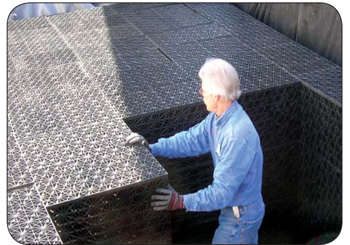
Underground outdoor systems can be customized to fit various shapes and sizes using these modular RainBoxes.
